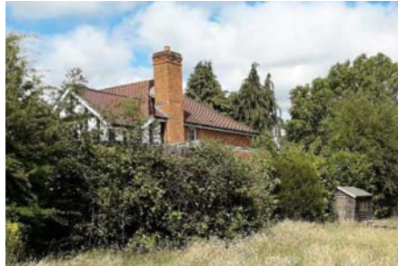
Looking at no. 4 from the application site
