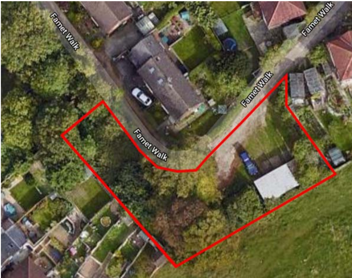
Fig 1: Existing site overview
